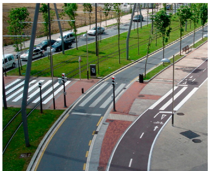
Figure 11: Four Modes, four different lanes – Mode separation for light rail, motorised traffic, cyclists and pedestrians. © Andrea Broadous, Bilbao, Spain, 2008
